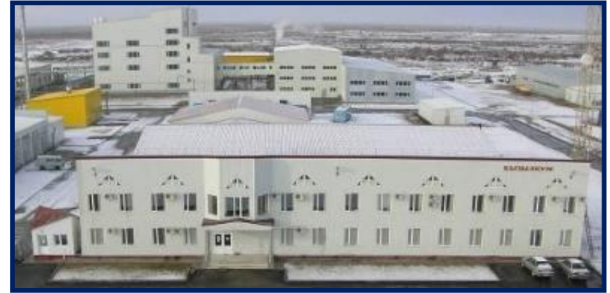
Processing facilities at Kharasan
