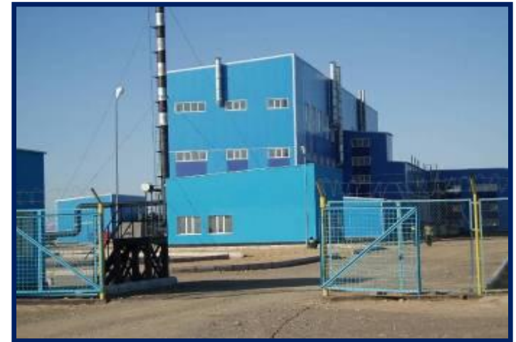
South Inkai production facilities
